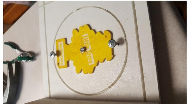
One more hurdle had to be cleared with the latest version of the Gilbertson PVC box. The new ones now have a PVC board as the roof, which lasts much longer than wood, but also is much denser and harder to insert a screw. The solution was to install a moly in the hole, screw through the scented tree and into the moly, problem solved.
